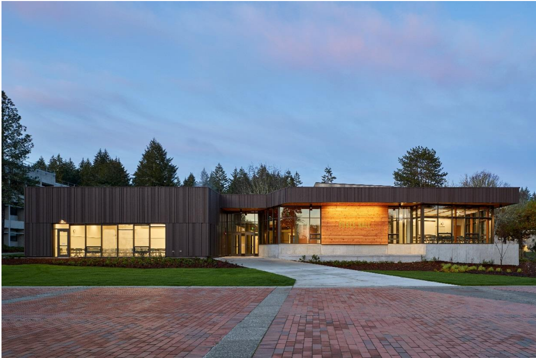
Purce Hall, a new lecture hall renovation on Evergreen’s Olympia campus. Courtesy of Evergreen.
